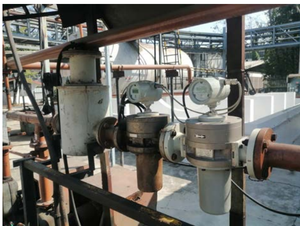
(L-R) – Diesel unloading point with master meter, Forklift filling area flowmeter, NHNT Testing cell inlet PD meter with master meter
