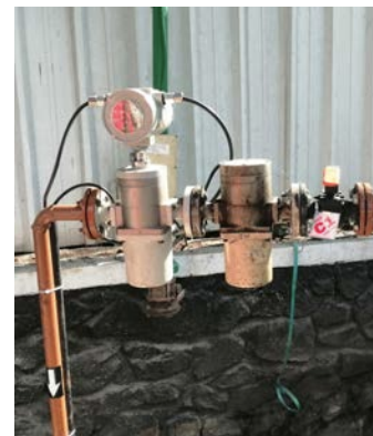
(L-R) – Diesel unloading point with master meter, Forklift filling area flowmeter, NHNT Testing cell inlet PD meter with master meter
