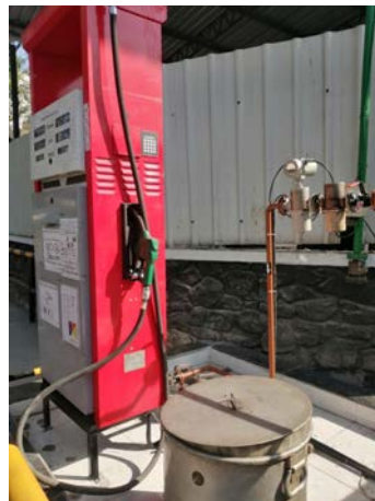
(L-R) – Diesel unloading point with master meter, Forklift filling area flowmeter, NHNT Testing cell inlet PD meter with master meter
